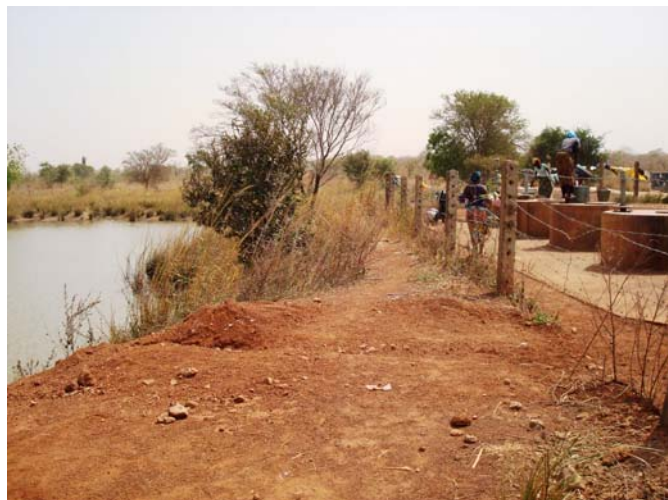
Figure 36 Gbrumani Dam and hand pumps, Tolon District
