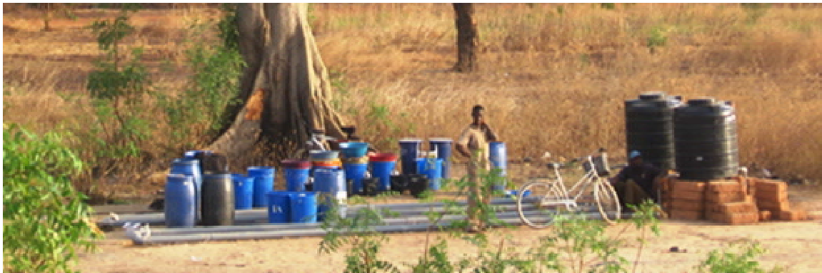
Figure 46 Ghanasco Dam HRF pilot system (January-February 2008)
