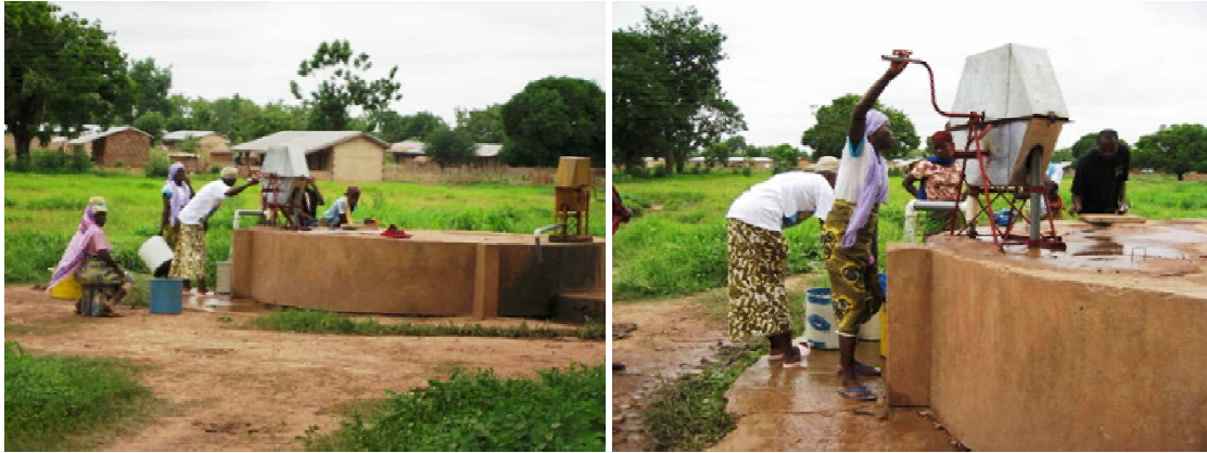
Figure 77 Cistern (left) and rope and washer hand pump (right) in the rainy season at Kunyevilla Dam, near Tamale, Northern Ghana Photo Credit: Kelly Doyle (2007)
