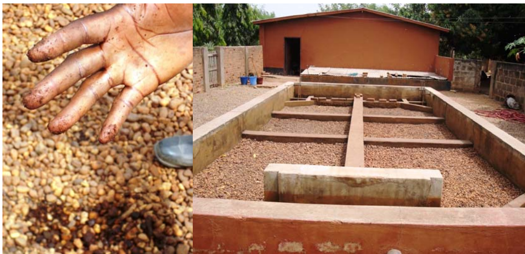
Figure 85 Mafi Kumase HRF: dirty gravel media (left) and view of HRF from the inlet (right)
