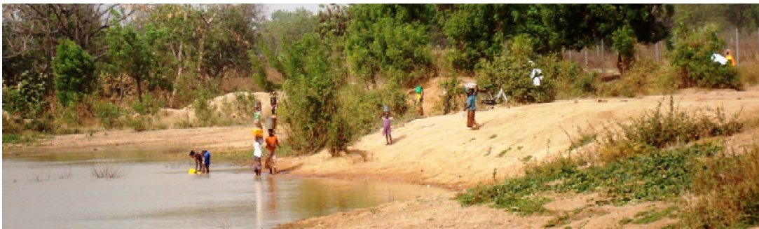
Figure 44 Ghanasco Dam, Tamale, Northern Region Ghana
