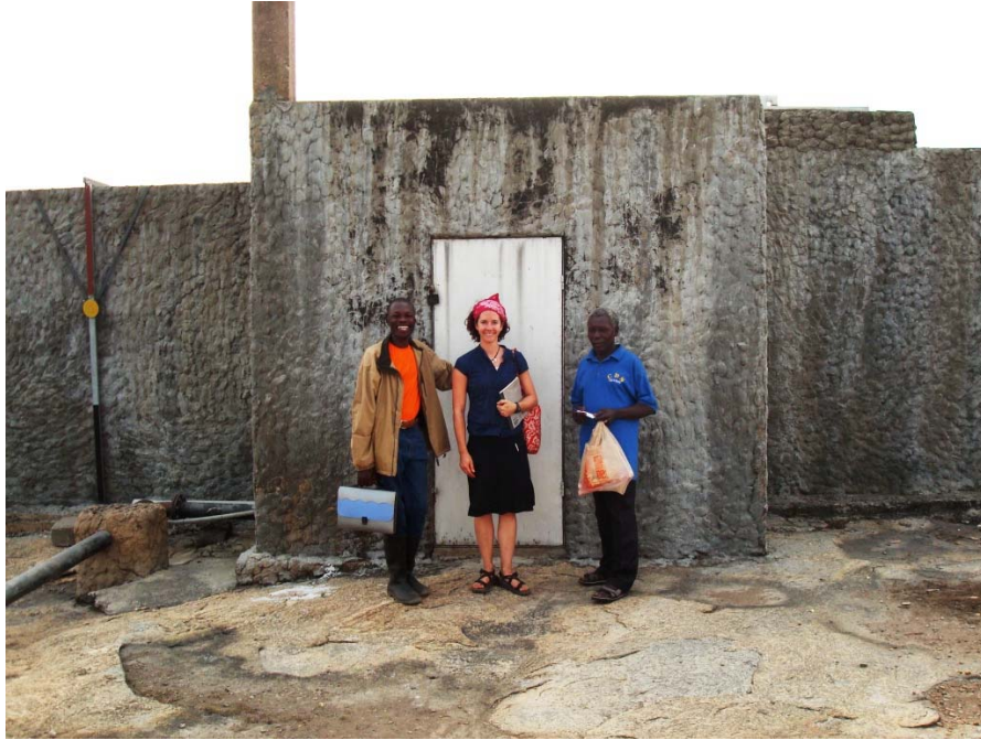
Figure 86 Perry, the author, and Dickens in front of the Mafi Kumase water tanks
