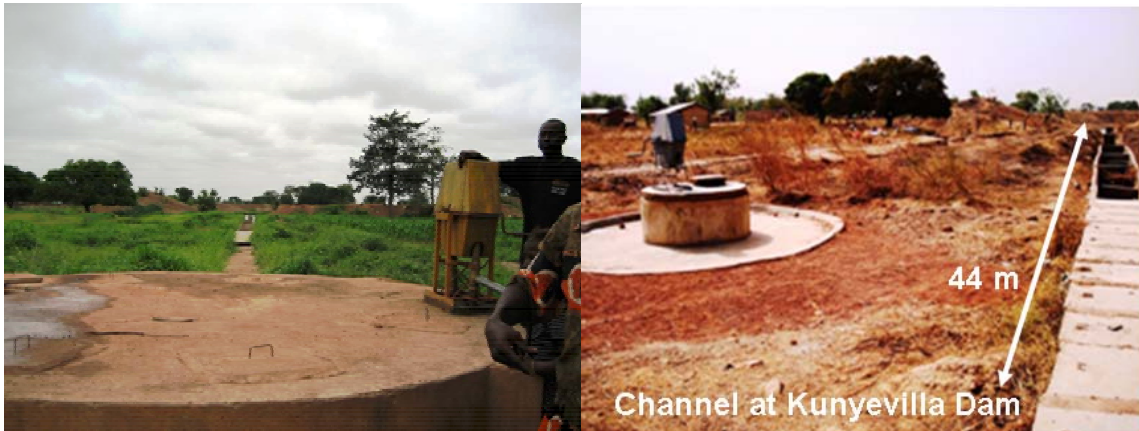
Figure 76 Kunyevilla Dam cistern and channel in the rainy season (left) and the dry season (right) Photo Credit: Kelly Doyle (2007) (left)
