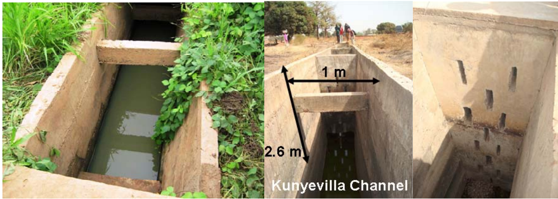
Figure 75 Kunyevilla Dam channel in the rainy season (left) and dry season (center and right) Photo Credit: Kelly Doyle (2007) (left)
