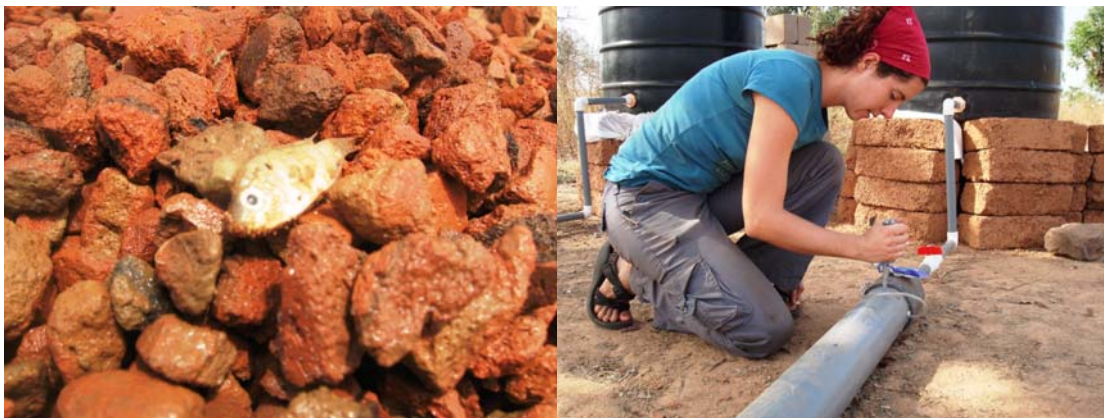
Figure 68 Pilot HRF maintenance: fish found in ceramic filter (P) (left) and author removing air bubbles (right)
